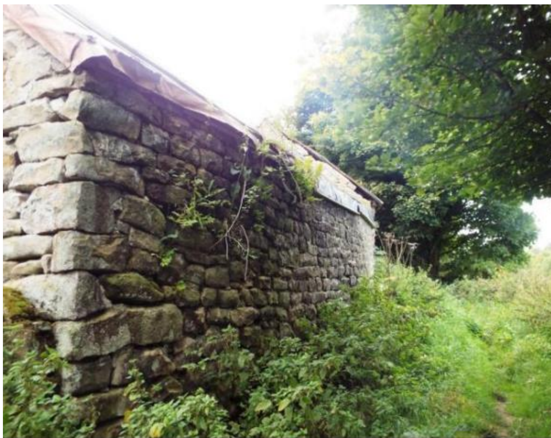
Figure 5 - Rear wall taken from 2015 structural survey, random stone brought to courses.
